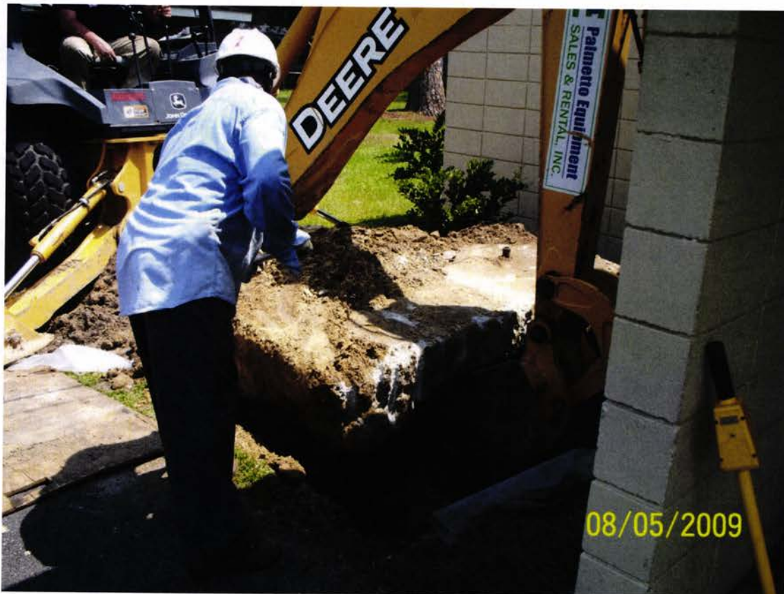
Picture 2: UST 1437Dove site during concrete ballast removal.
